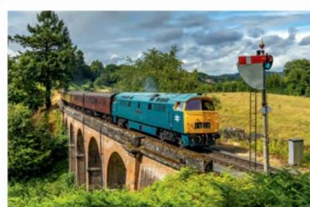
The Western Locomotive Association's immaculate Class 52 diesel-hydraulic D1062 Western Courier crosses Oldbury Viaduct on the Severn Valley Railway, working the 15.35 Bridgnorth to Kidderminster service on July 6 during the SVR's 1940s Weekend. Kevin Whitehurst
