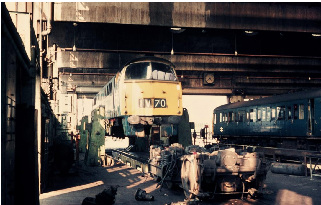
D1038 Western Sovereign is seen on the jacks at Laira TMD in August 1970.
