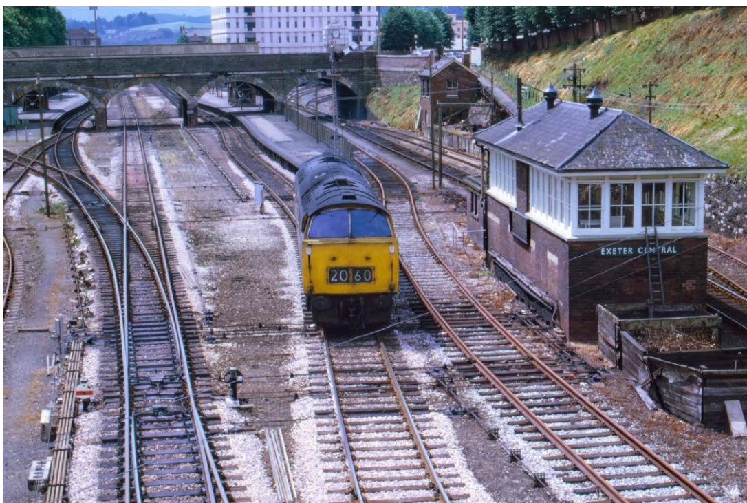
D1052 Western Viceroy at Exeter Central at 13.58 on 16 th July.
